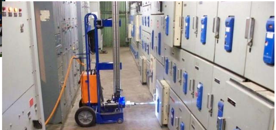
Remote racking system
