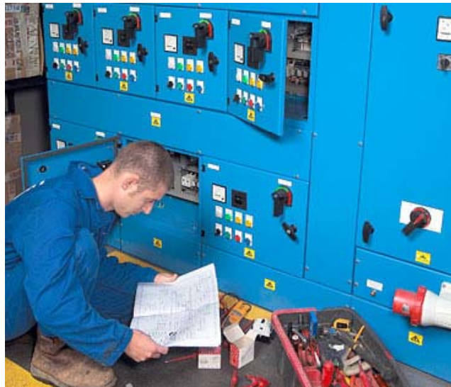
Safety related maintenance requirements
